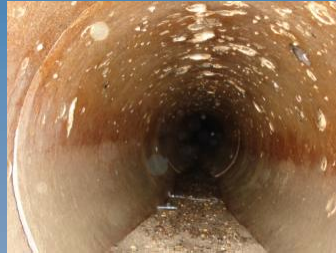
Approximately 18 miles of pipe for MSANK sewer system
